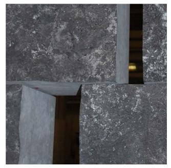
The wall is necessarily massive. Though capable of being an inertia wall the individual blocks are dowelled together to form a continuous framework. No opening at the lower level is greater than 100mm. The "rear" and sides of the stones have a sawn finish revealing the fossils buried in the stone. Though unpolished the stone reveals this secret when wet.
